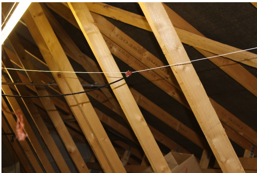
Loft mounted 6m wire dipole at G4BCA's QTH
